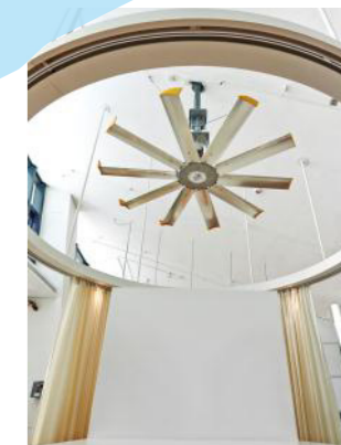
Figure 3.3.11 High Volume Low Speed (HVLS) fan (Source: Construction Industry Council)
