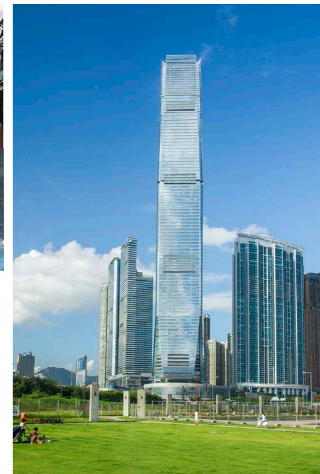
Figure 3.2.31 Exterior of International Commerce Centre (Source: Kai Shing Management Services Limited)
