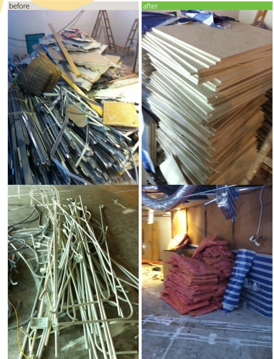
Figure 3.1.60 Construction and demolition waste were sorted (Source: Hong Kong Green Building Council)
