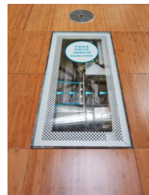
Figure 3.3.10 Under floor cooling (Source: Construction Industry Council)
