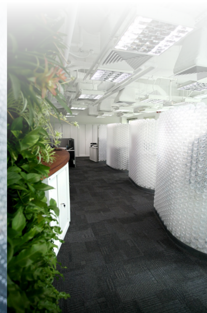
Figure 3.2.27 POLLI-BRICKS Wall as Partition Wall (Source: Hong Kong Green Building Council)
