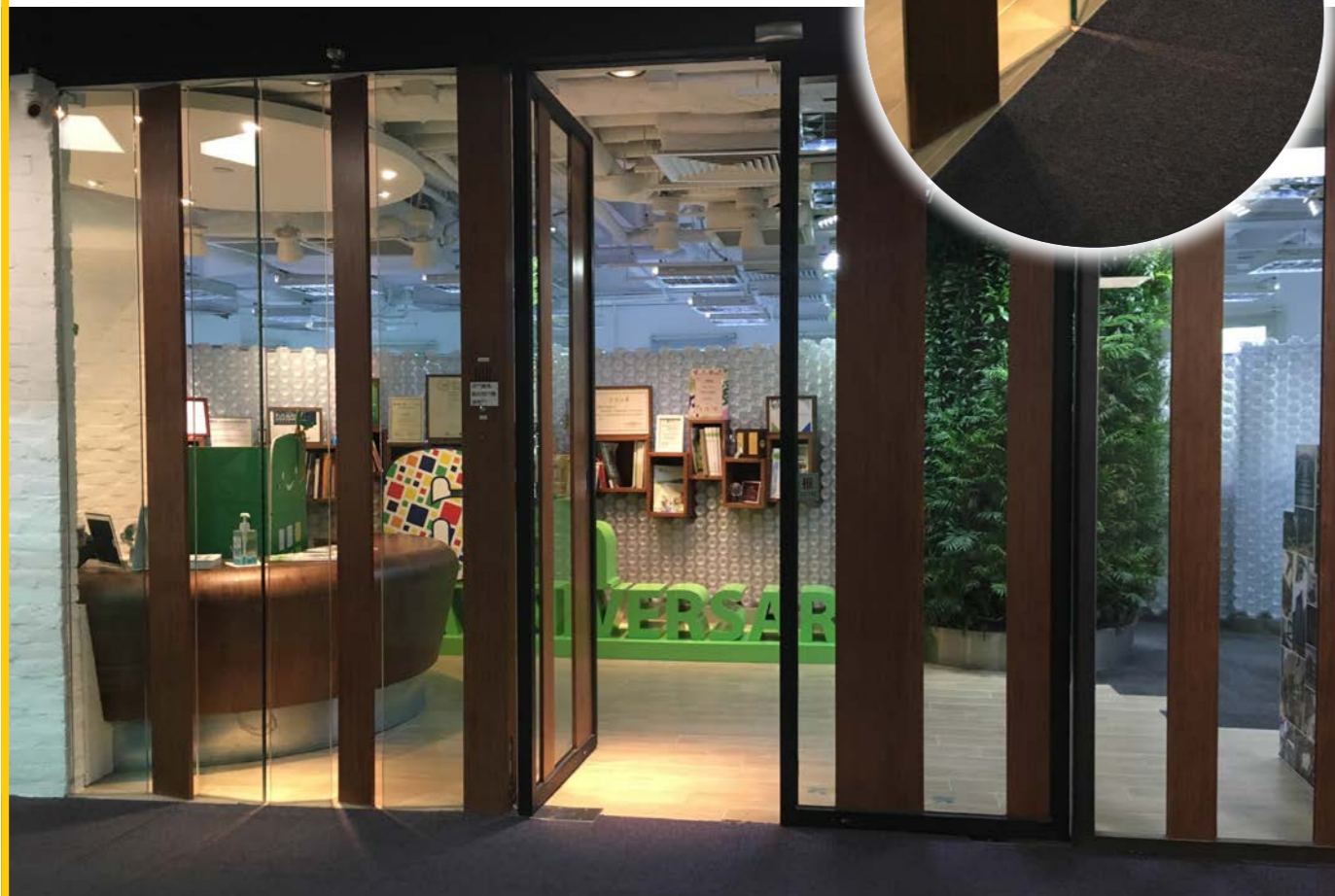
Figure 3.2.14 Louvered wall at main entrance (Source: Hong Kong Green Building Council)
