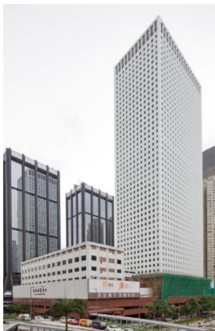
Figure 3.1.53 Original China Resources Building (Source: China Resources Property Limited)
