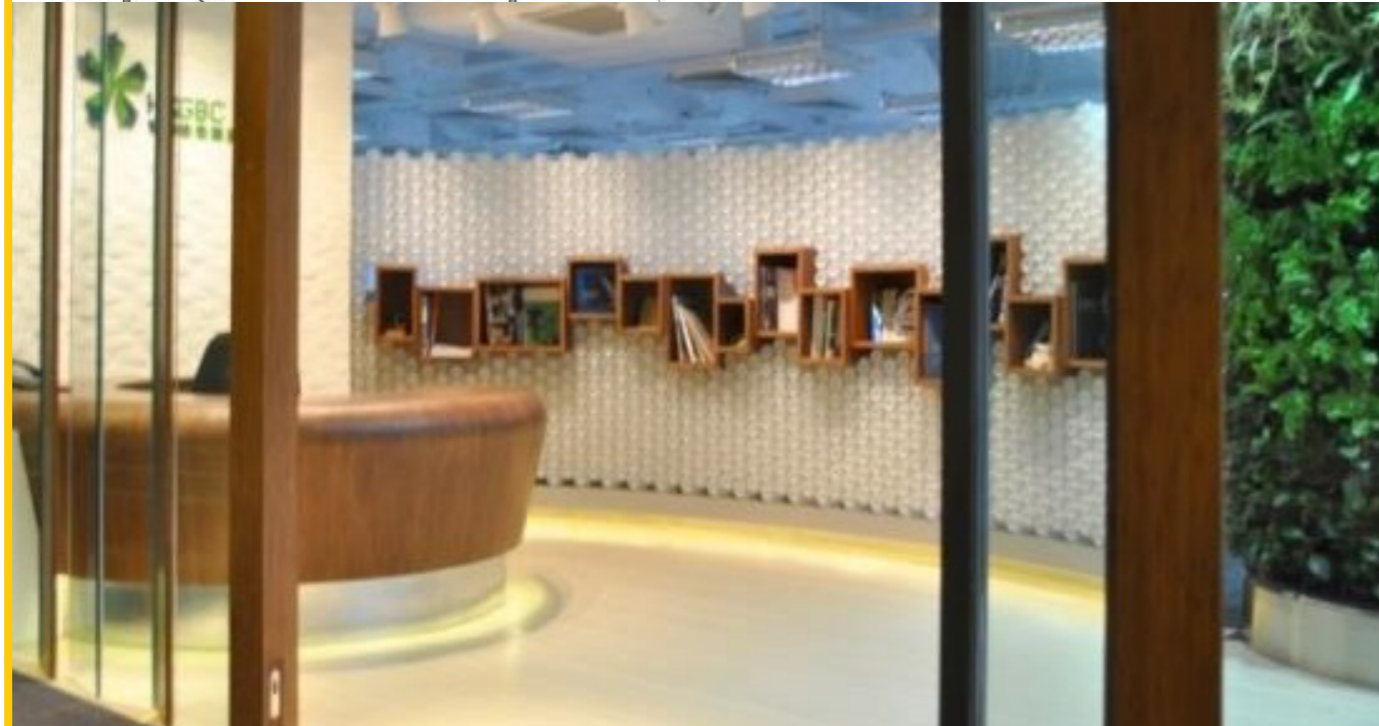
Figure 3.2.36 Hong Kong Green Building Council louvered wall for ventilation (Source: Hong Kong Green Building Council)
