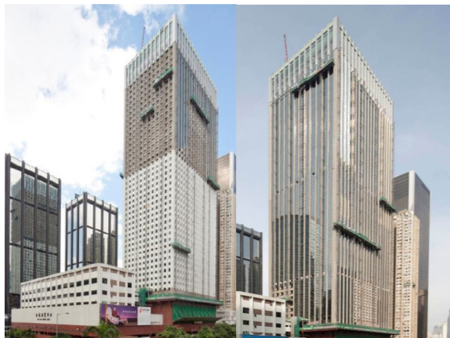
Figure 3.1.54 China Resources Building under construction (Source: China Resources Property Limited)
