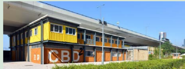
Figure 5.15 Energizing Kowloon East Office (Source: Energizing Kowloon East Office)
