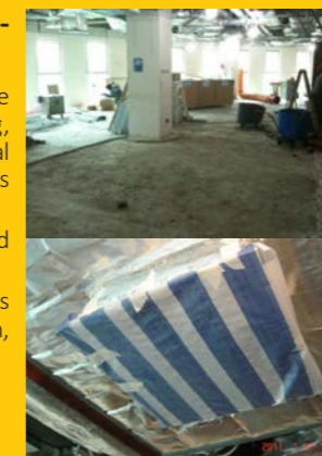
Figure 3.1.56A Protection to existing air duct
