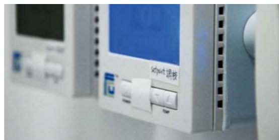
Figure 3.2.4 Electronic thermostat for individual control (Source: Hong Kong Green Building Council)
