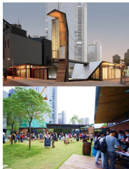
Figure 4.1.7 Sha Tin Community Green Station (Environmental Protection Department) (Source: Press release of news.gov.hk (11 May 2015), “Sha Tin Community Green Station open to public from tomorrow”, available at http://www.info.gov.hk/gia/general/201505/11/P201505110596.htm )
