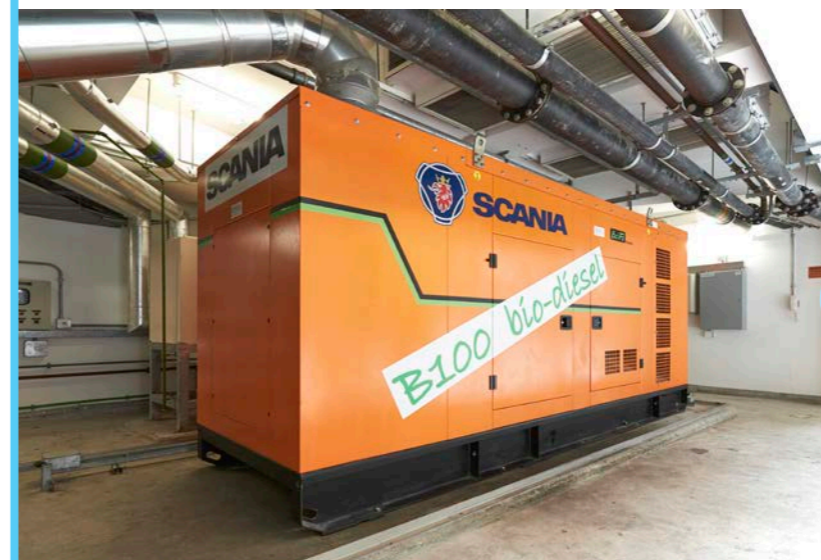
Figure 3.3.2 Bio-diesel Tri-generation (Source: Construction Industry Council)
