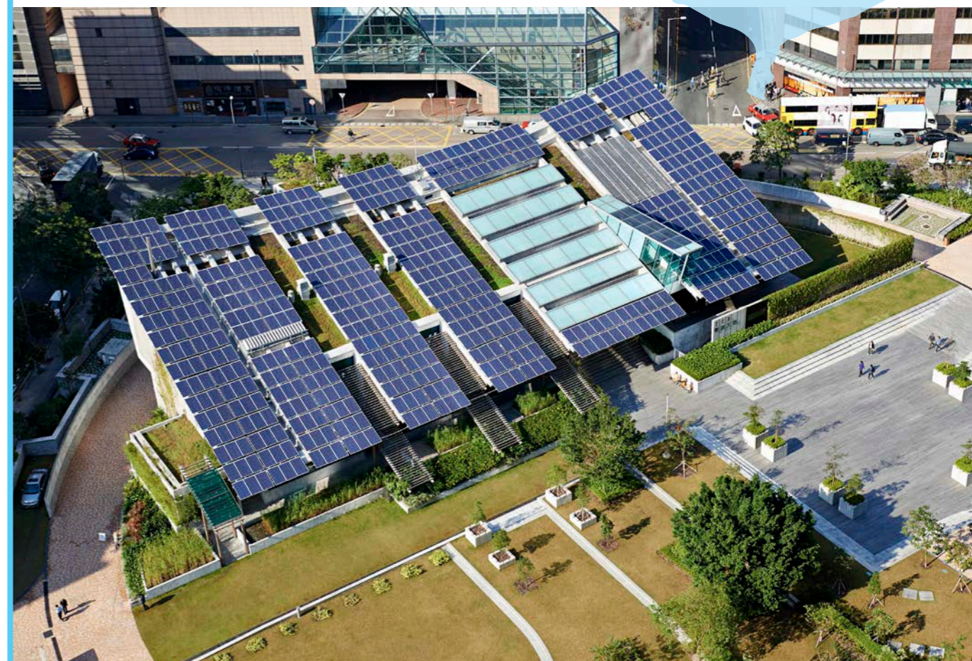
Figure 3.3.3 Solar Panel of Zero Carbon Building (Source: Construction Industry Council)
