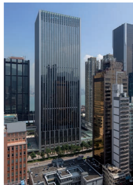
Figure 3.1.55 China Resources Building after renovation (Source: China Resources Property Limited)
