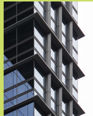
Figure 3.2.19 Glare control (Source: Hysan Development Company Limited)
