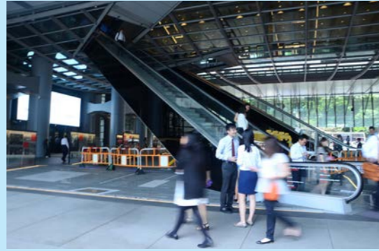
Figure 3.1.4 Ground Connection at HSBC Headquarter
