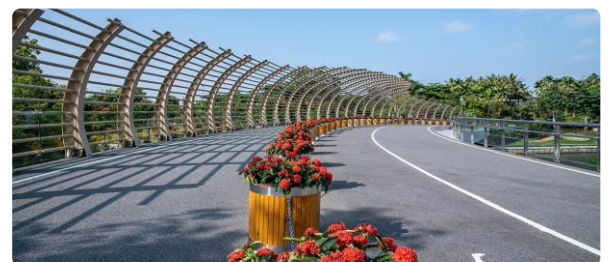
Figure 26: Shenzhen Bay Sports Park – Coastal Runway and Bicycle Lanes
