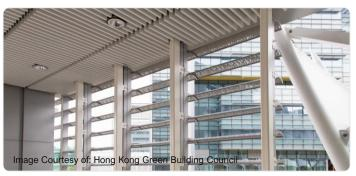
**Figure 54: Thermostat-actuated Louvres** Solar tracking louvres to maximise ventilation and insulate western sun in Hong Kong Science Park Phase 3.
