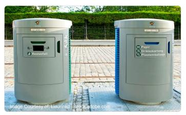
Figure 70: Sustainable Waste Management Mechanisms Waste bins in Norway integrated with a pneumatic waste collection system.
