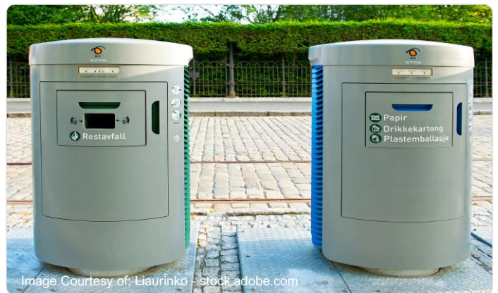
Figure 70: Sustainable Waste Management Mechanisms Waste bins in Norway integrated with a pneumatic waste collection system.
