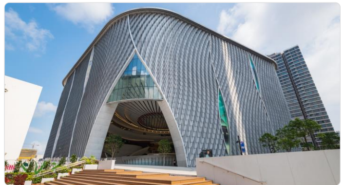
Figure 53: Consideration of Building Facades Curved metal fins on the exterior façade of Hong Kong’s Xiqu Centre act as shading devices to reduce heat gain and energy consumption.
