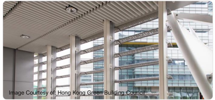
Figure 54: Thermostat-actuated Louvres Solar tracking louvres to maximise ventilation and insulate western sun in Hong Kong Science Park Phase 3.
