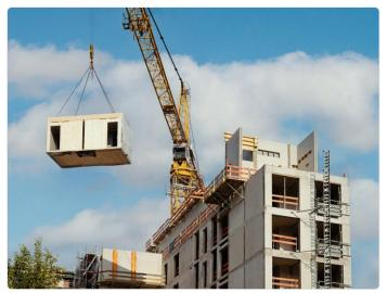
Figure 99: Adoption of MiC Lifting and installation of MiC modules on construction site.
