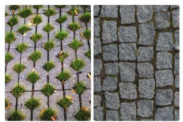
Figure 50: Sustainable Drainage Systems Concrete grid pavers (left) and natural rock pavers (right).
