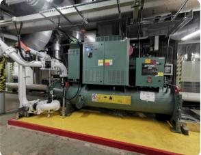
Figure 143: High Efficiency Night Load Chiller
