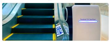
Figure 110: Surface Disinfection UV steriliser for escalator handrails.
