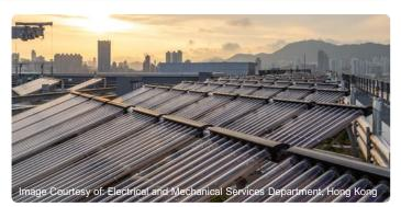
Figure 60: Rooftop PV Panel Installation Solar Water Heating Systems at Hong Kong Children's Hospital.
