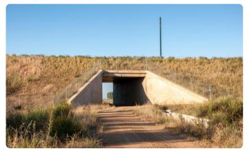
Figure 82: Incorporate Wild-Life Design Illustration of a wildlife corridor at a high-speed railway. Wildlife can cross the railway through the corridor without the risk of roadkill.
