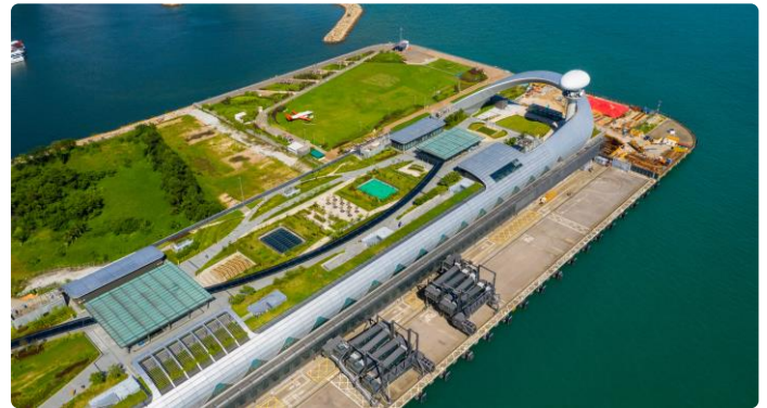
Figure 80: Identify Opportunities for Green/Blue Infrastructure Green roof adopted at the Kai Tak Cruise Terminal building in Hong Kong.
