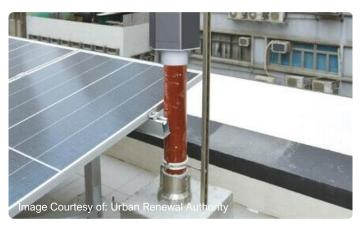
**Figure 115: Regular Maintenance of Existing Buildings** A simulation of a UVC sterilisation device installed on a rooftop ventilation pipe by the URA.
