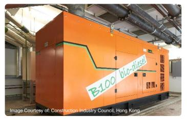
**Figure 71: Electricity Generation via Biofuel** Use of biodiesel tri-generation system at CIC-Zero Carbon Park to generate electricity from biofuel made of used cooking oil.
