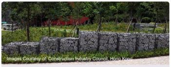
Recycled debris salvaged from demolition waste used for gabion walls
