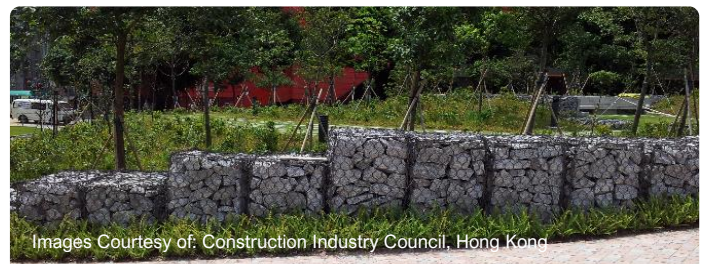
Recycled debris salvaged from demolition waste used for gabion walls
