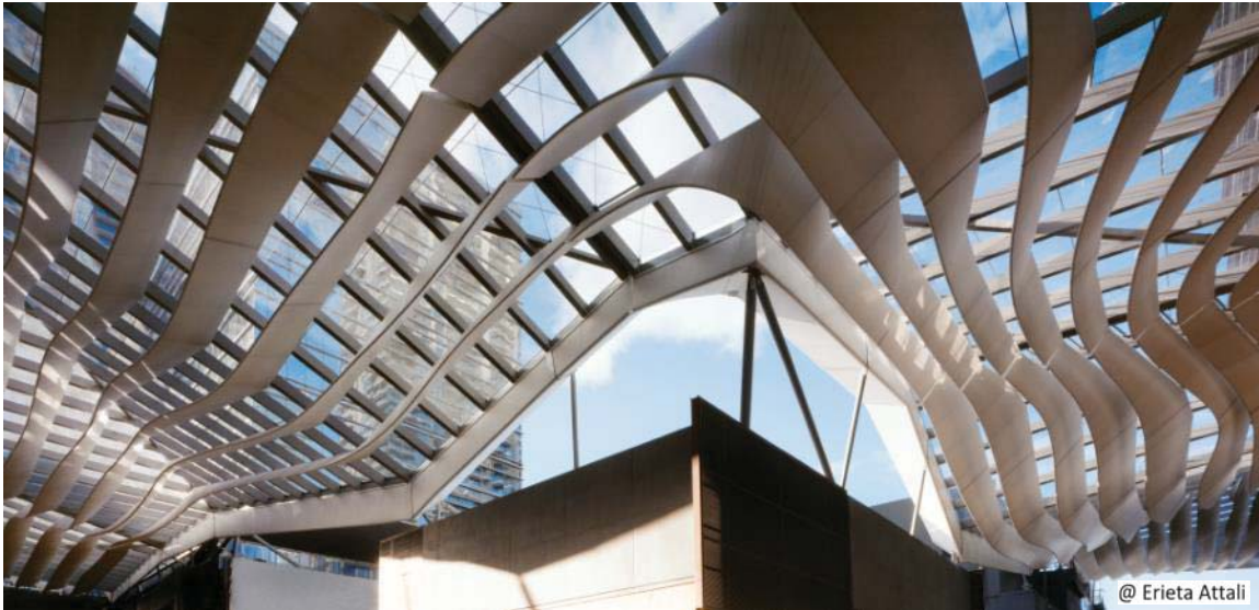
Figure 4: A 100,000 sq ft faceted canopy of steel and glass undulates between the mall, hotel, offices and residential towers
