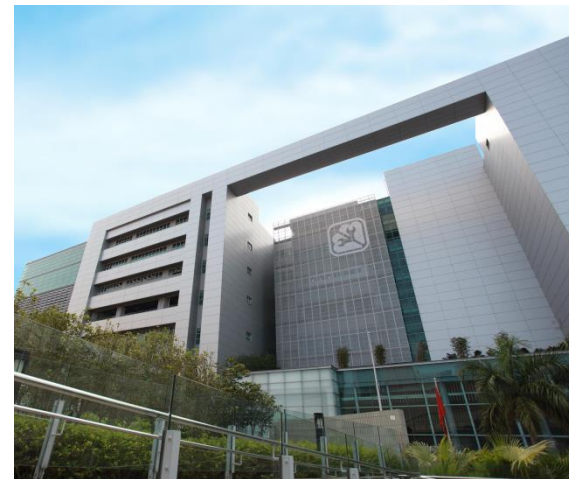
Electrical and Mechanical Services Department Headquarters Existing Buildings V1.2 Final Platinum
