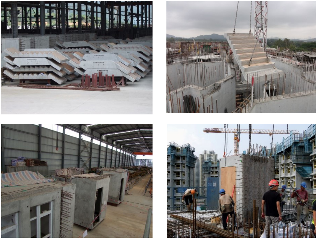
Figure 18 Examples of typical precast components used in the public residential buildings [HKHA, 2017]
