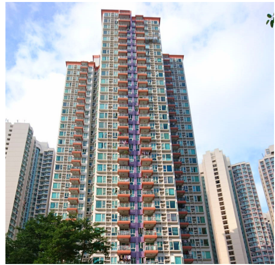
Figure 20 Fu Tei project in Tuen Mun achieved the cost-effectiveness by utilising precast structural components
