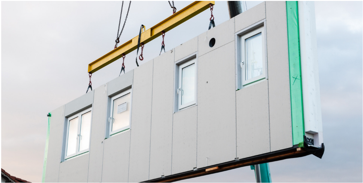
Figure 52 Use of prefabricated building components in construction sites
