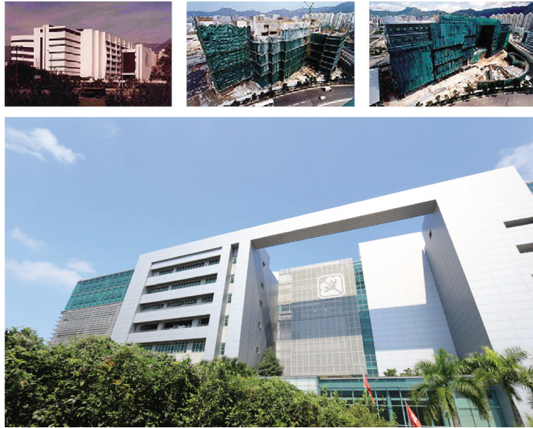
Figure 42 Retainability application on demolition project – EMSD Headquarters
