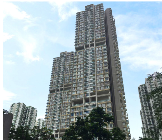
Figure 19 The Orchards adopted prefabrication which dramatically reduced more than half of the waste.
