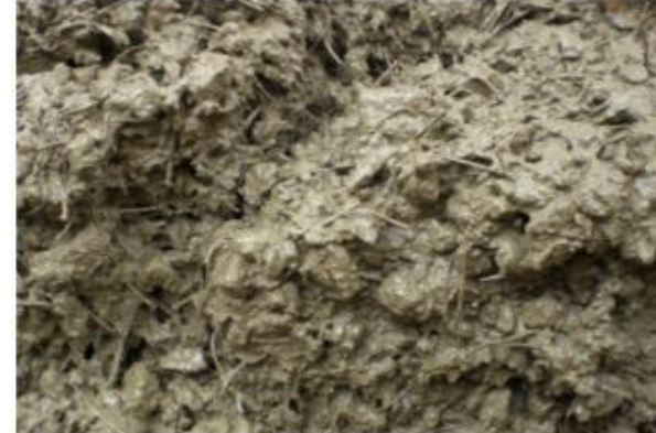
Close up of concrete composition
