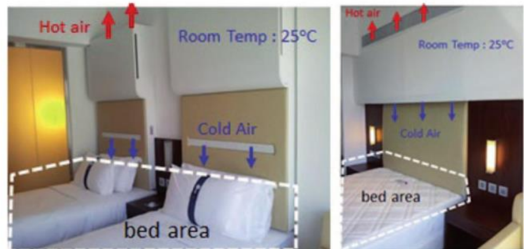
Fig. 7.10 Principle of operation of the Peltier headboard
