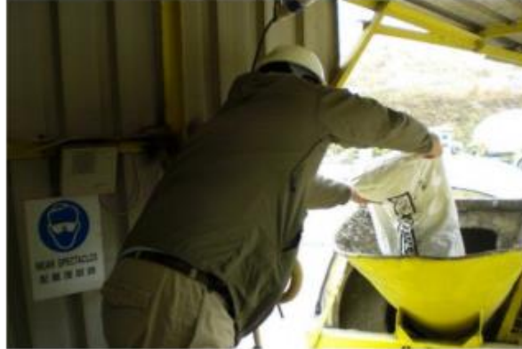
Adding fibers into revolving drum
