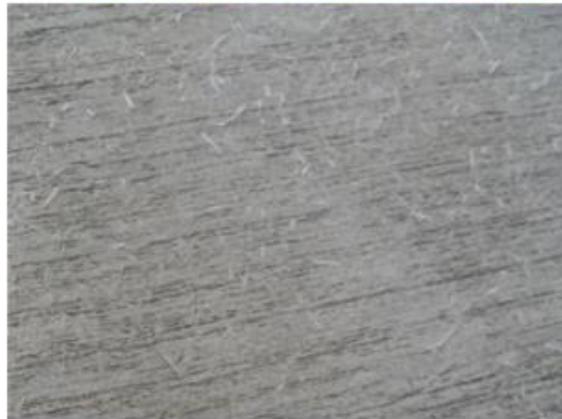
Profile of broom finished surface
