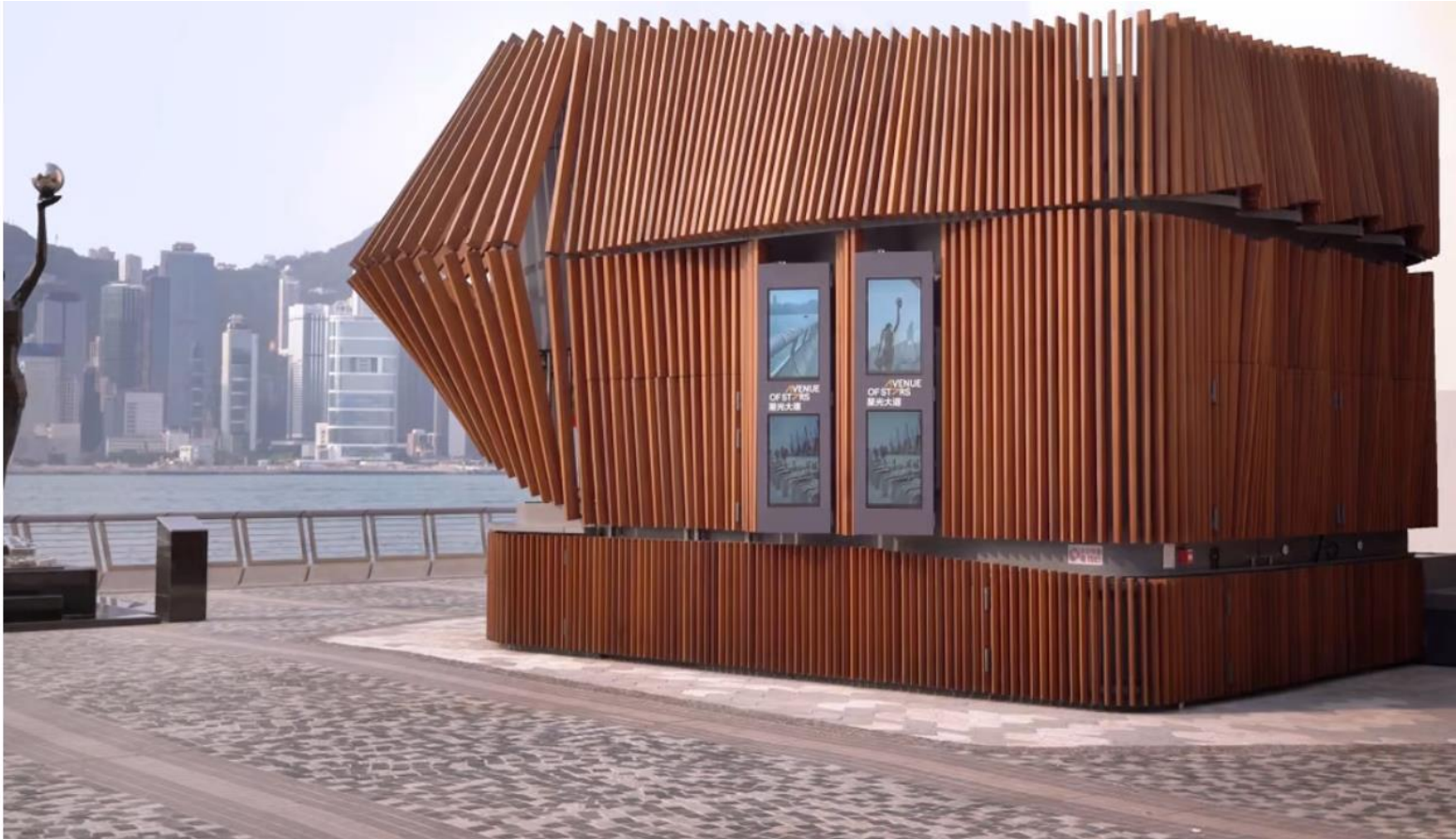
Hong Kong studio LAAB designed a food kiosk, called Harbour Kiosk, on the Avenue of Stars on the Tsim Sha Tsui promenade, made out of red balau wood.
