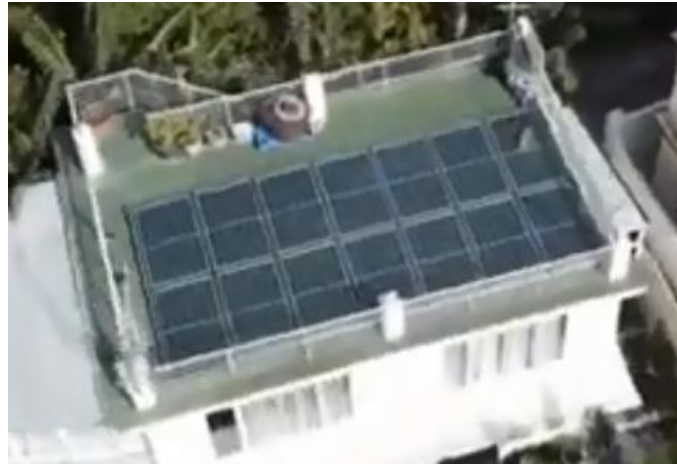
Walkable PV panels laid as floor tiles
